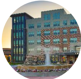
The Residences at Annapolis Junction
